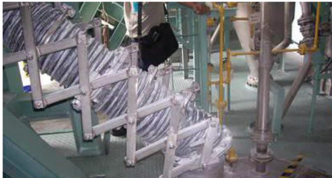
3Star Fabric Expansion Joint ducting specially designed with Pantograph Frame and Liner for PIA transfer from Truck to Storage Tank, during operation, the Expansion Joint accepts very large axial motion and the pantograph allows equal movement for every section of a fabric expansion joint
